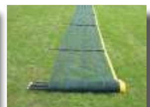
5. Roll up fencing with poles in place.
