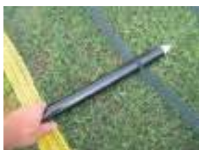
1. Insert poles into fencing.
