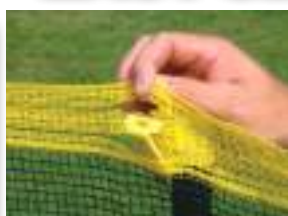
2. Attach fence to top cap.
