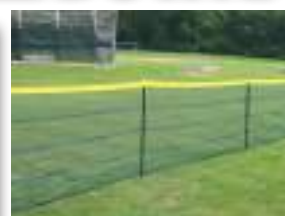
4. Place poles & sockets in holes.
